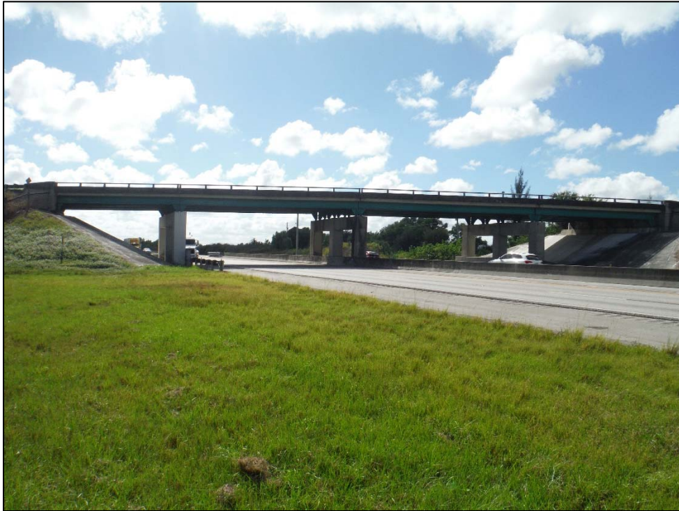
Figure 22: FDOT Bridge No. 940050 (8SL3282) over Florida's Turnpike, facing Southwest
