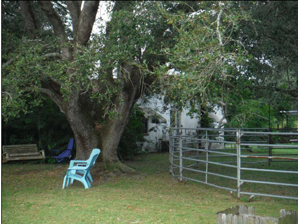
Figure 18: House located at 4362 W. Midway Road (8SL1806), facing Northwest
