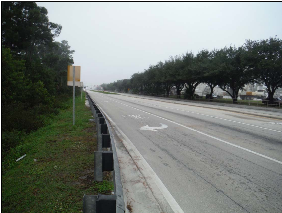
Figure 17: Midway Road (8SL1657) from East of Torino Parkway, facing Northwest
