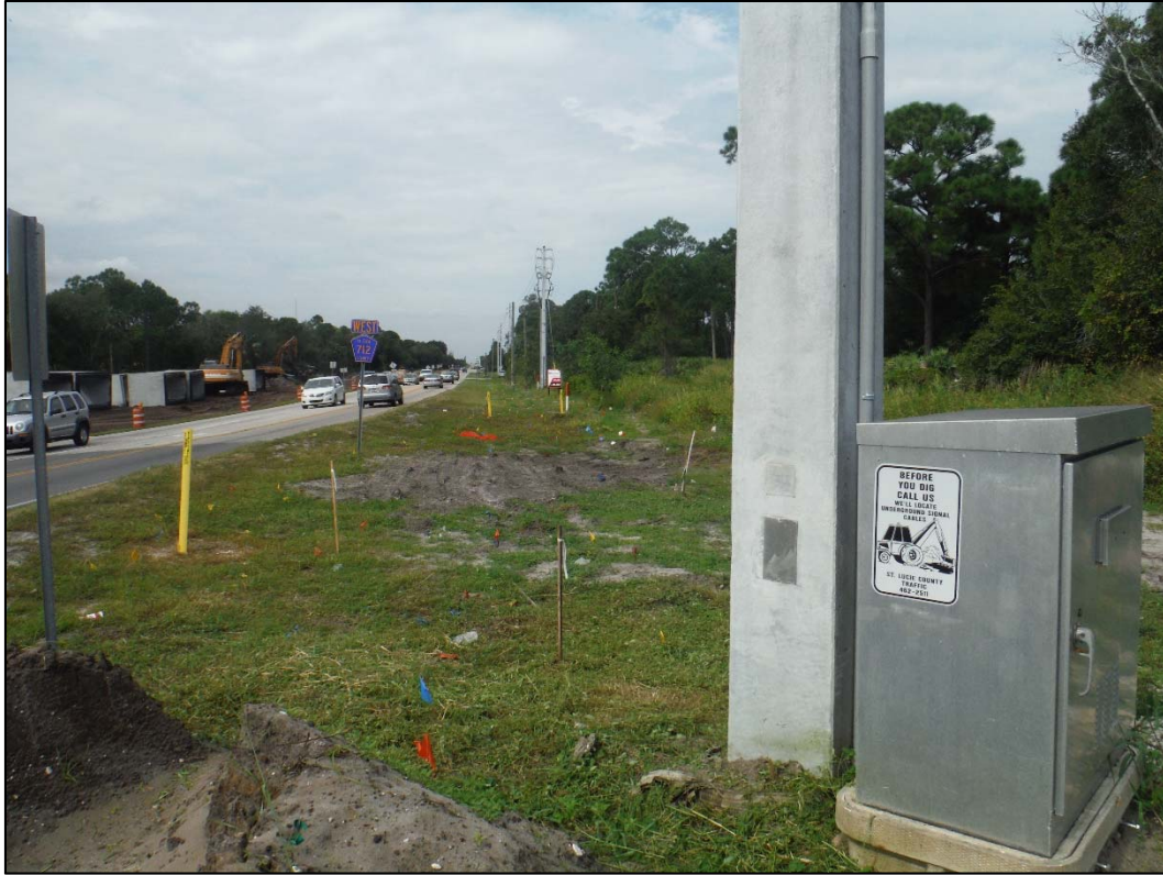
Figure 12: Project Area West of Selvitz Road with Buried Utilities, facing West
