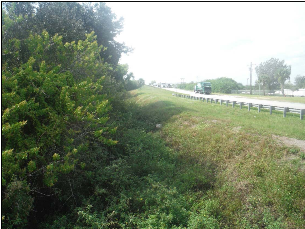
Figure 20: Canal 103 (8SL1809) from NW Corporate Way, facing West
