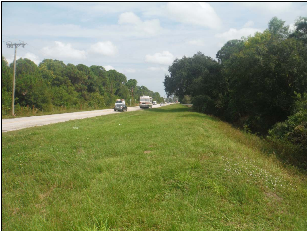
Figure 11: Project Area South of Midway Road with Canal and Spoil Berm, facing East
