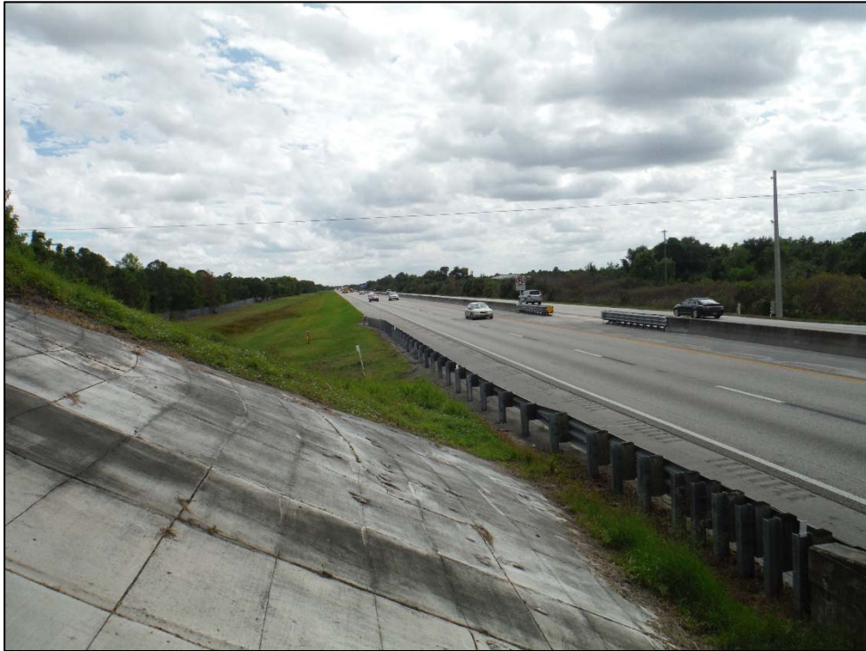
Figure 10: Florida's Turnpike from Beneath FDOT Bridge No. 940050, facing Southeast
