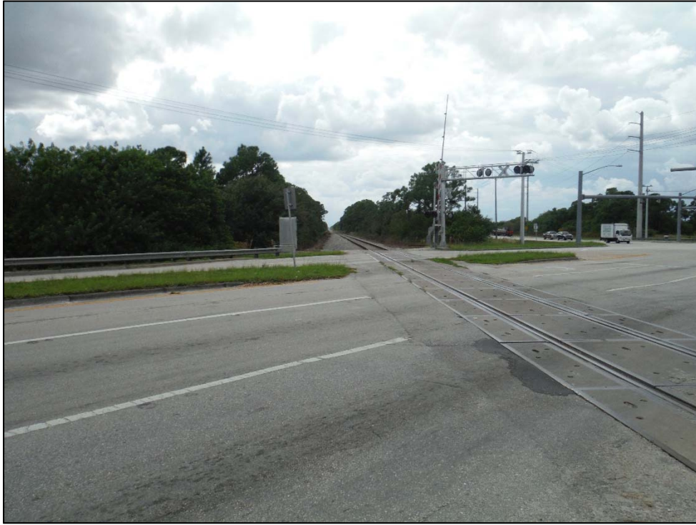
Figure 16: FEC Railroad – Lake Harbor Branch (8SL3014) Tracks at Intersection with Midway Road in APE, facing Southwest
